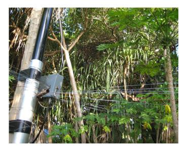
The good thing about running the radials in the bush is that when you do the work you can also pick up some papaws for the breakfast. At one moment I almost lost the telescopic mast in a heavy wind when an unidentified beast has eaten one of the guying ropes... had to replace guying ropes with zinc coated wire segments.
